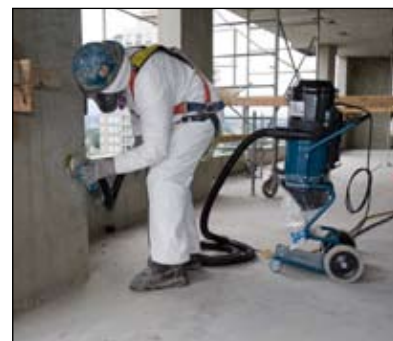
Worker grinding concrete using local exhaust ventilation
