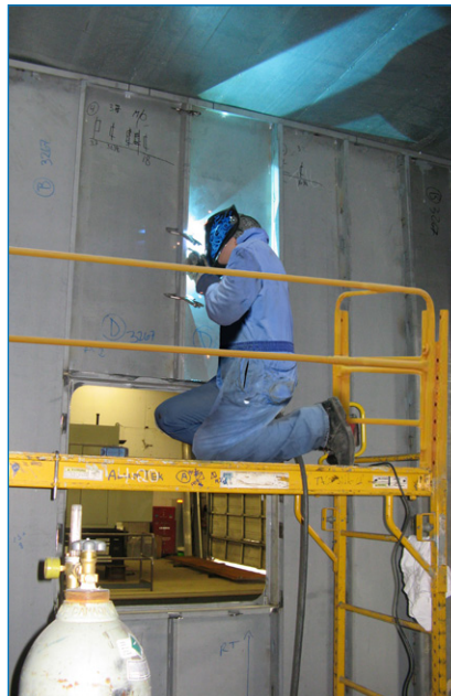
Use scaffolds to provide a raised working surface.
